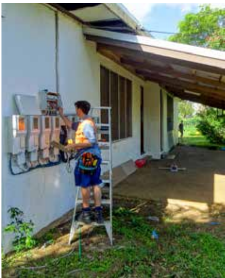
Cam busy connecting power to each unit to test his work.
