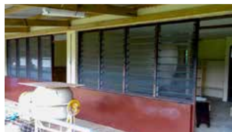
The outside of each unit with fixed louvres and new fly screens.
